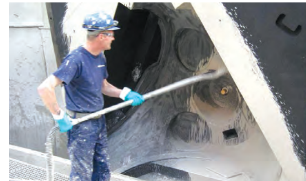
Flow coating application
