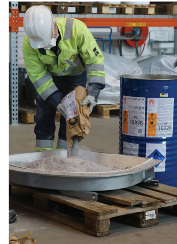
INITEK ISO granular refractory lining installation and exothermic set
