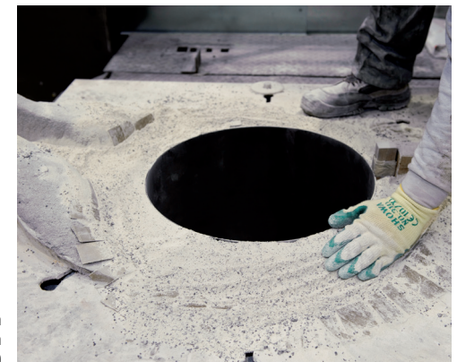
Coreless induction furnace lined with KELLUNDITE 400
