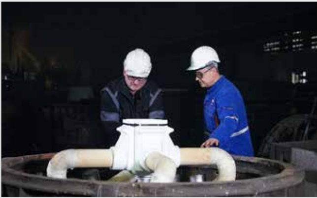
Fig. 5a: Filter box and running system installation in drag
