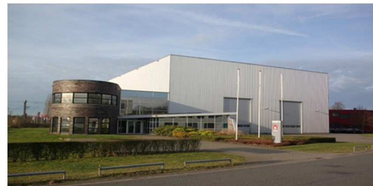
Foundry R&D facility, Enschede
